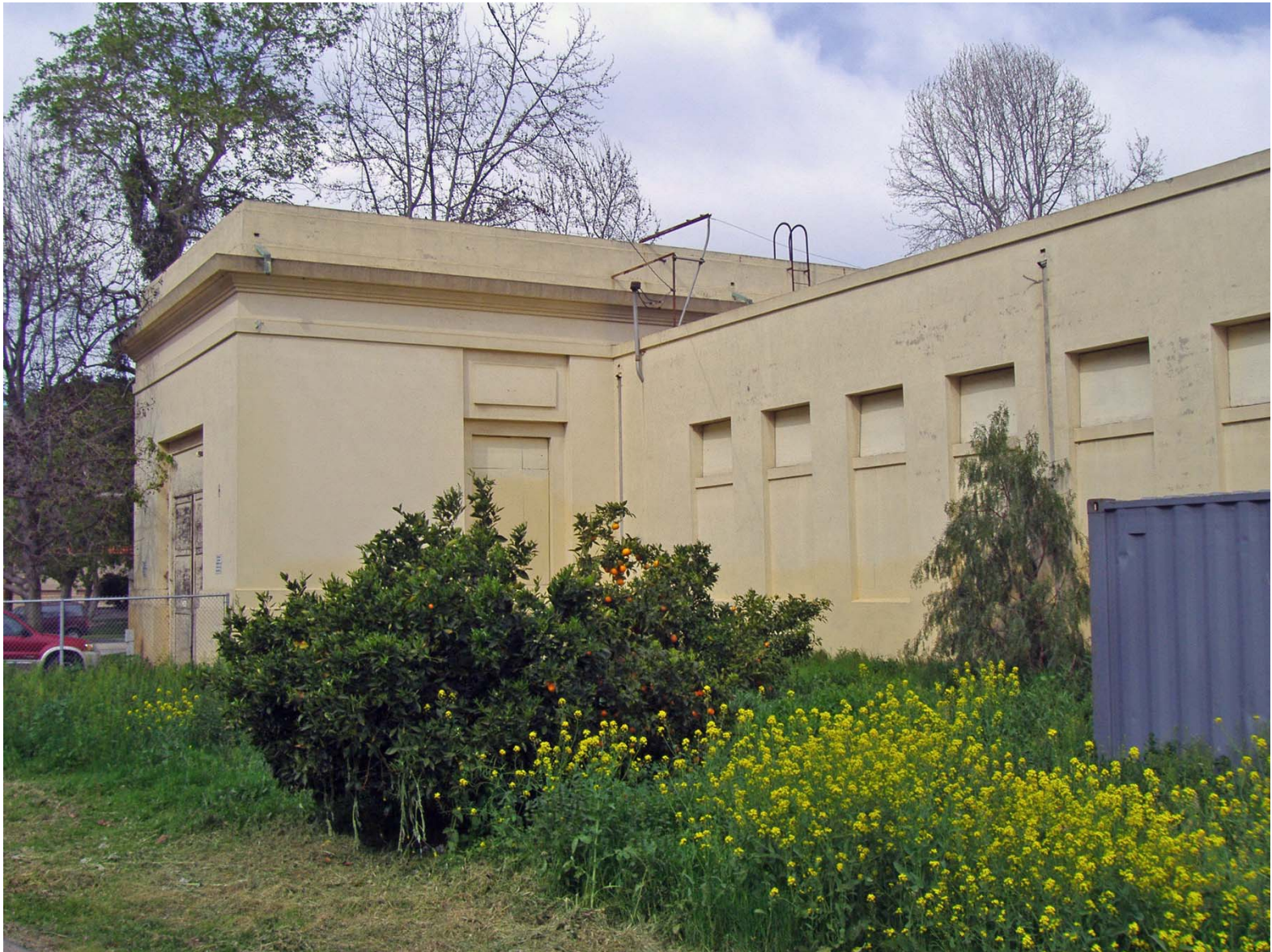
Overview of SD G & E Building (facing West/Northwest).
