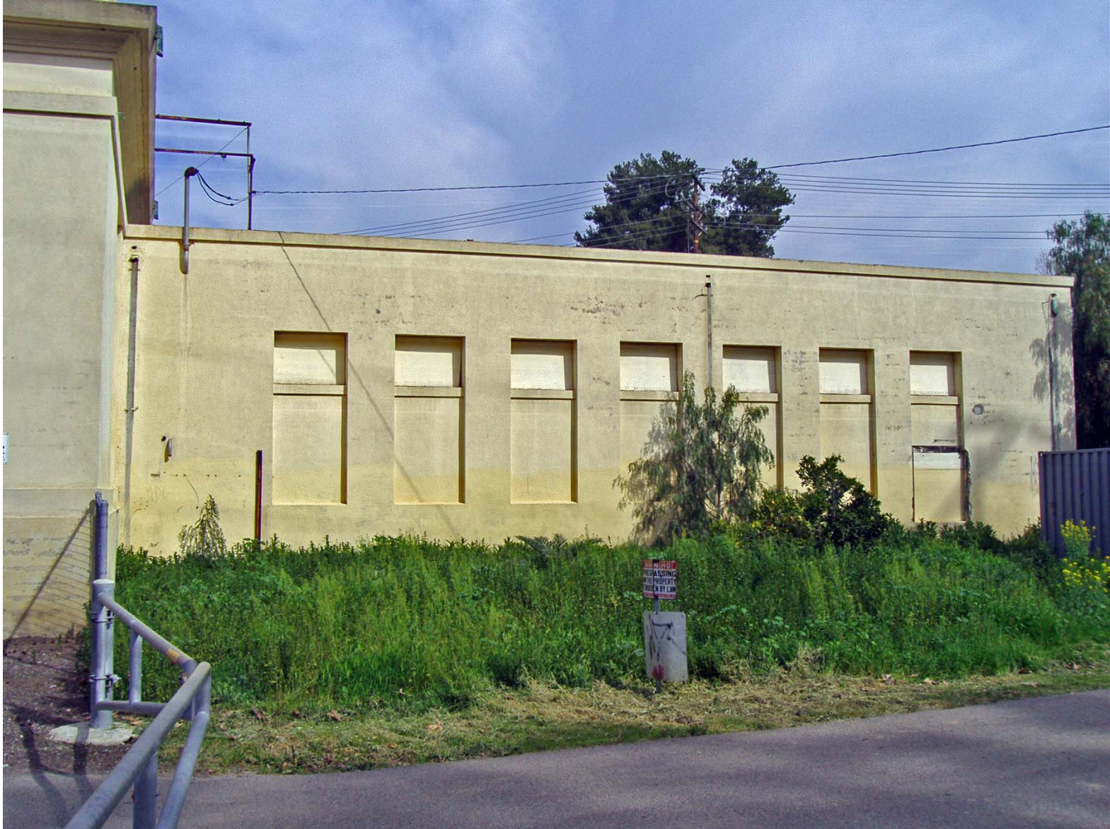
Overview of South Elevation fo Ell (with Altered Window; facing North).
