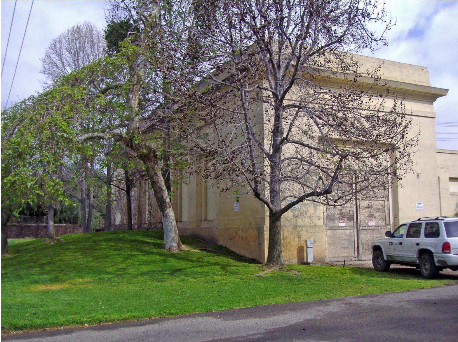
Overview of SD G & E Building from Southwest (facing Northeast).
