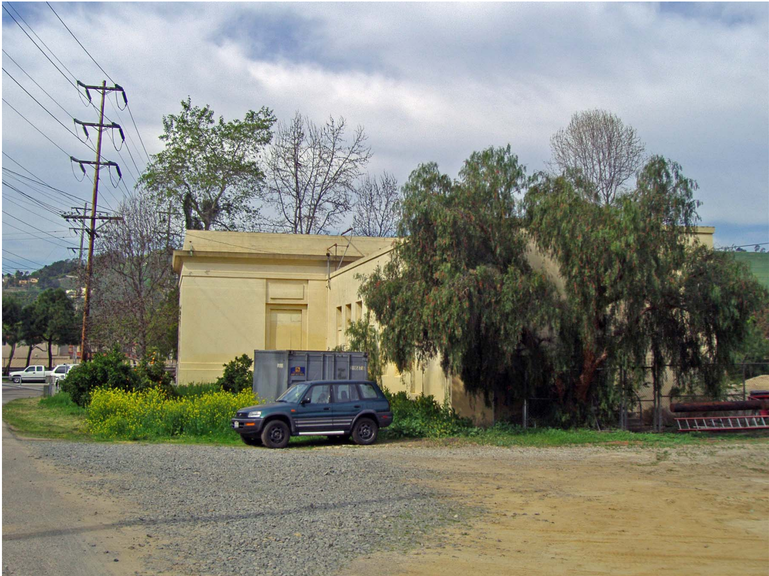
Overview of SD G & E Building from East (facing West/Northeast).
