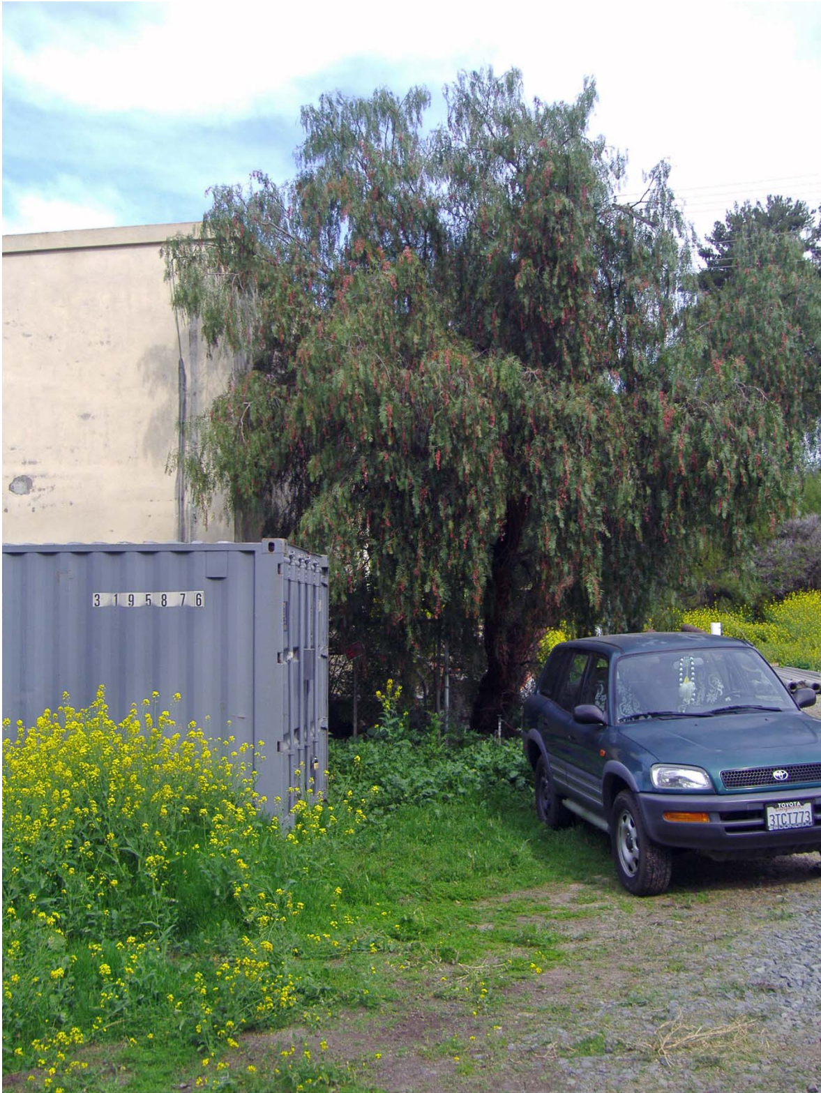
Overview of South Elevation from Southeast (Facing North).
