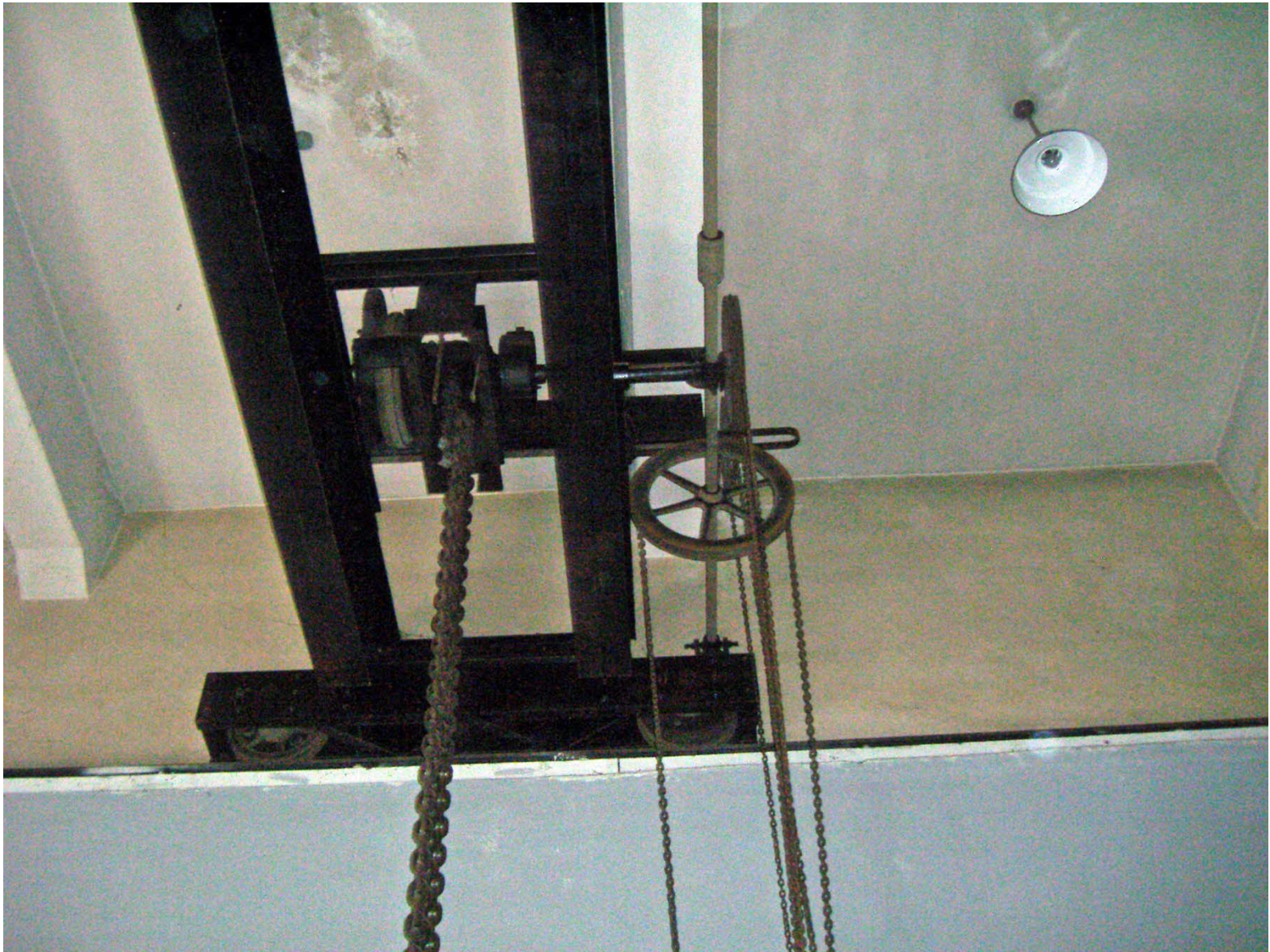
Detail of Crane Pulley System and Tracks along Wall (facing East).
