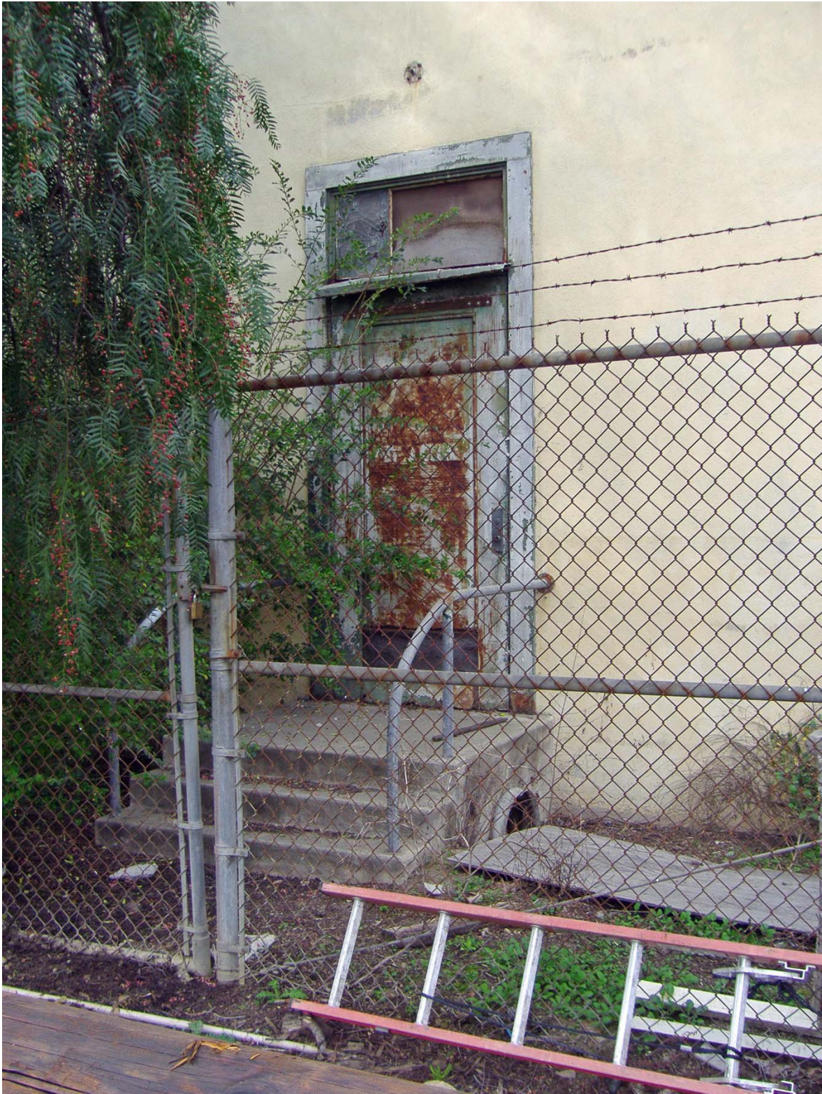
Rear Entry on East Elevation of E11 (facing Southwest).
