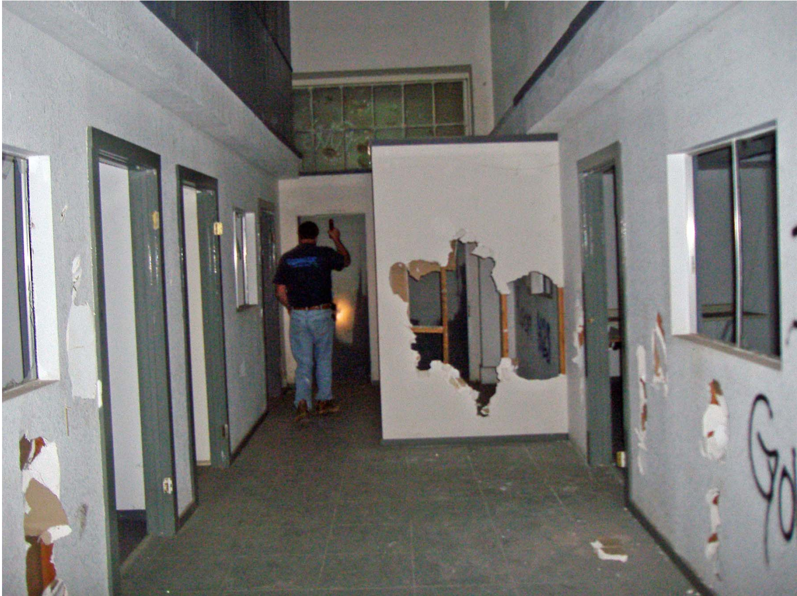
Interior of East Ell Illustrating Offices and Additional Walls (facing West).
