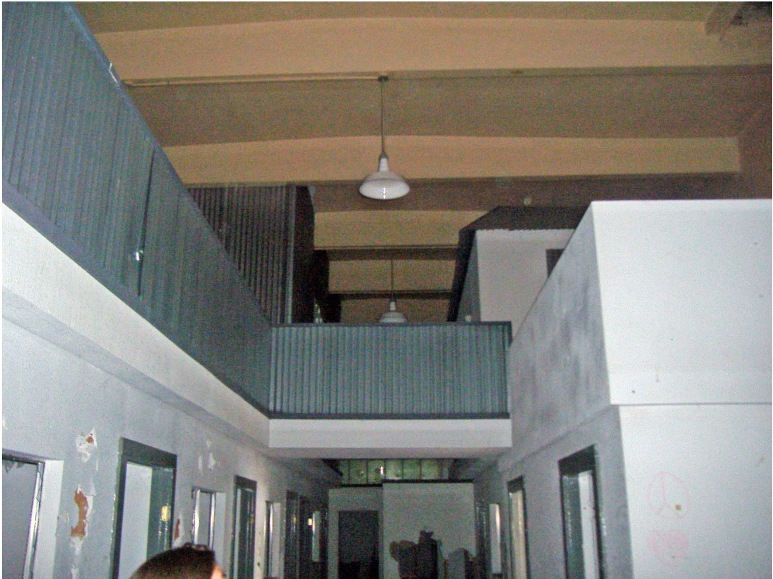
Overview of Secondary Offices and Ceiling Beams (facing West).
