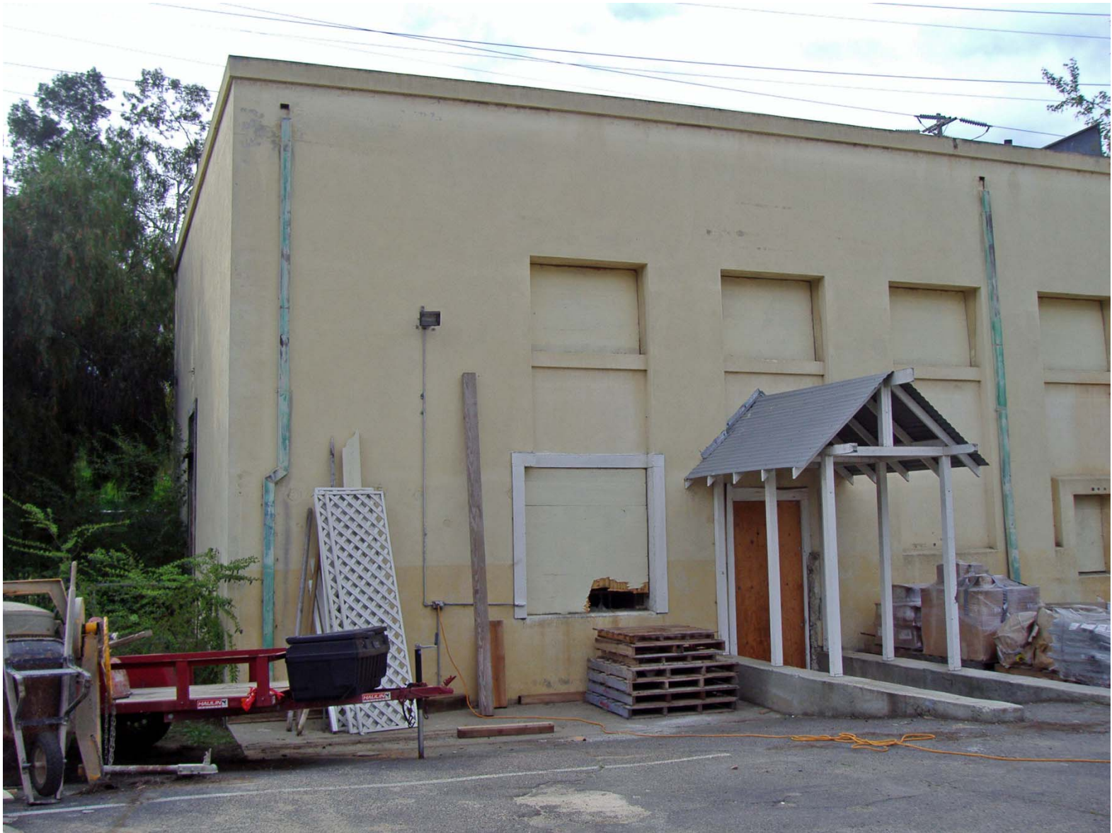
Overview of North Elevation of Ell with Altered Window and Added Covered Doorway (facing South).
