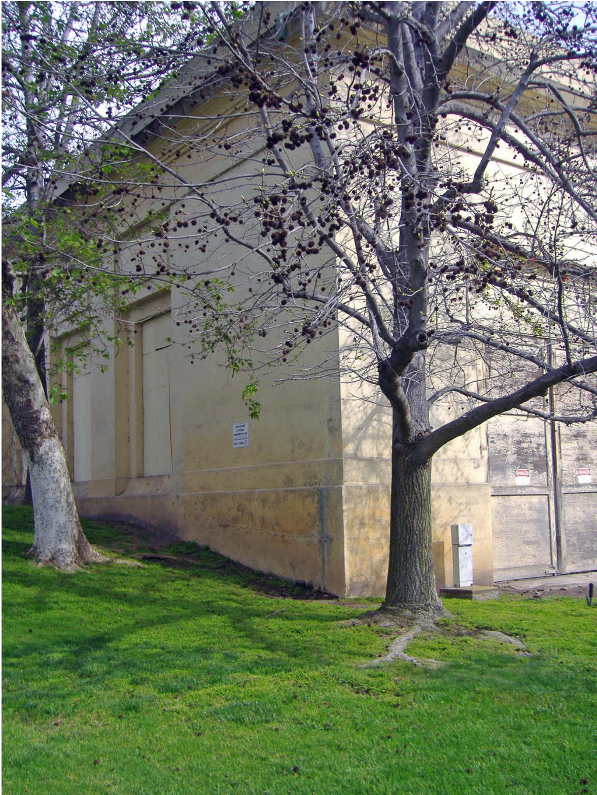
Overview of Southwest Corner of SD G & E Building (facing Northeast).
