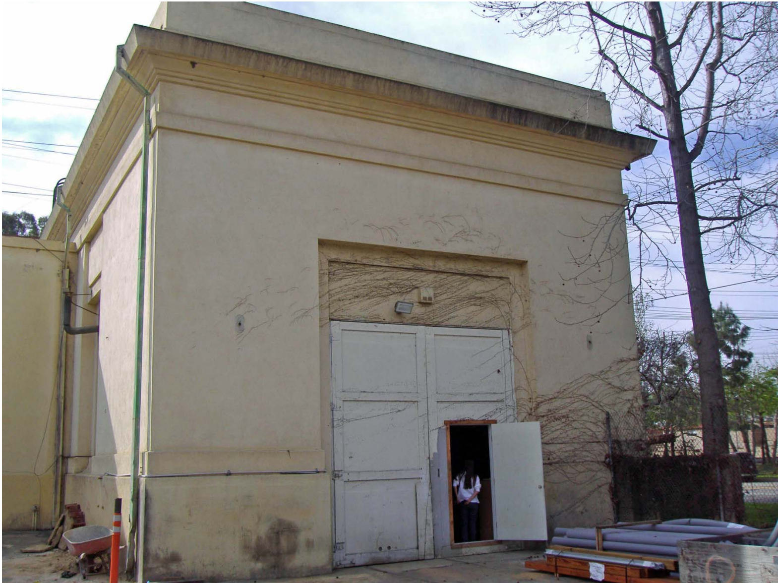
Overview of North Elevation of SDG & E Building (facing South/Southwest).
