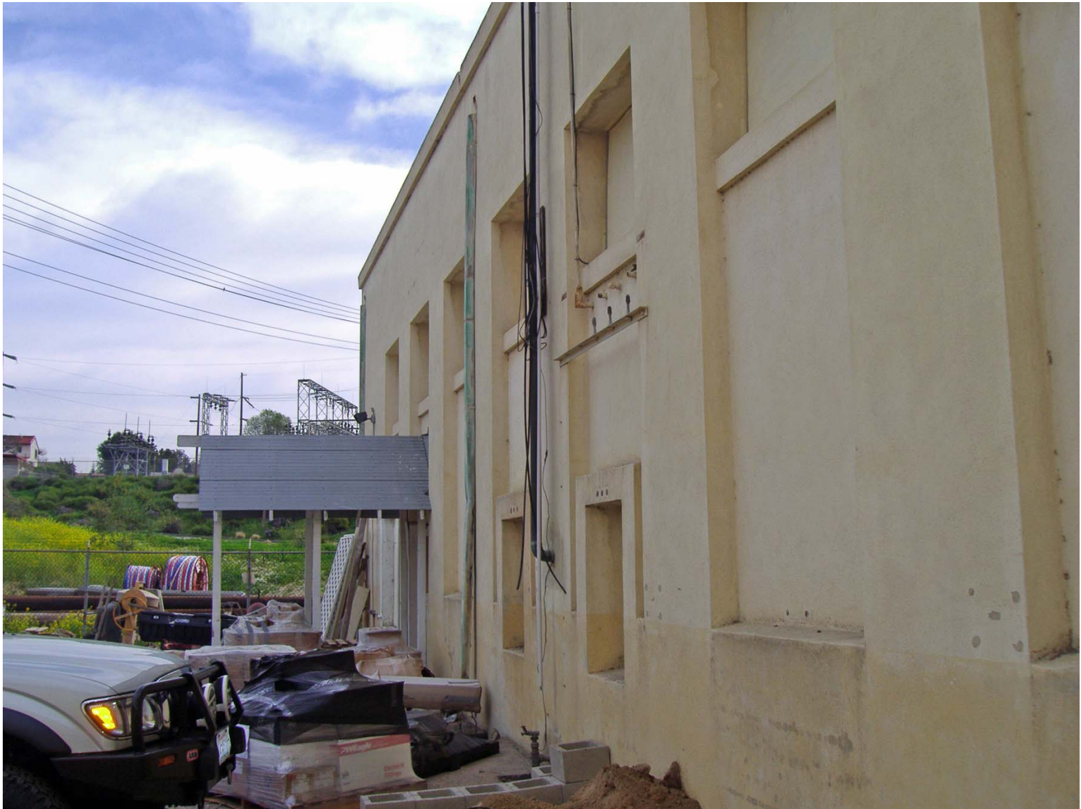
Overview of North Elevation fo East Ell (facing East/Southeast).
