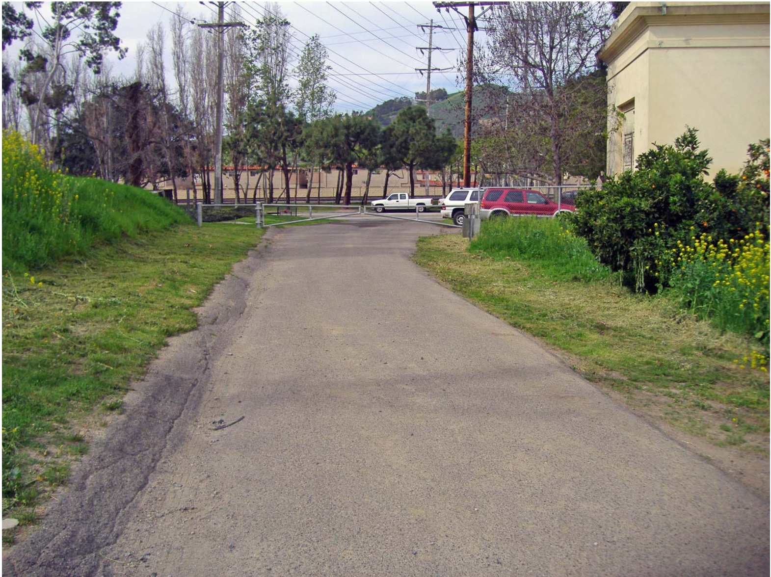
Overview of Main Drive at Camino Capistrano (facing West).
