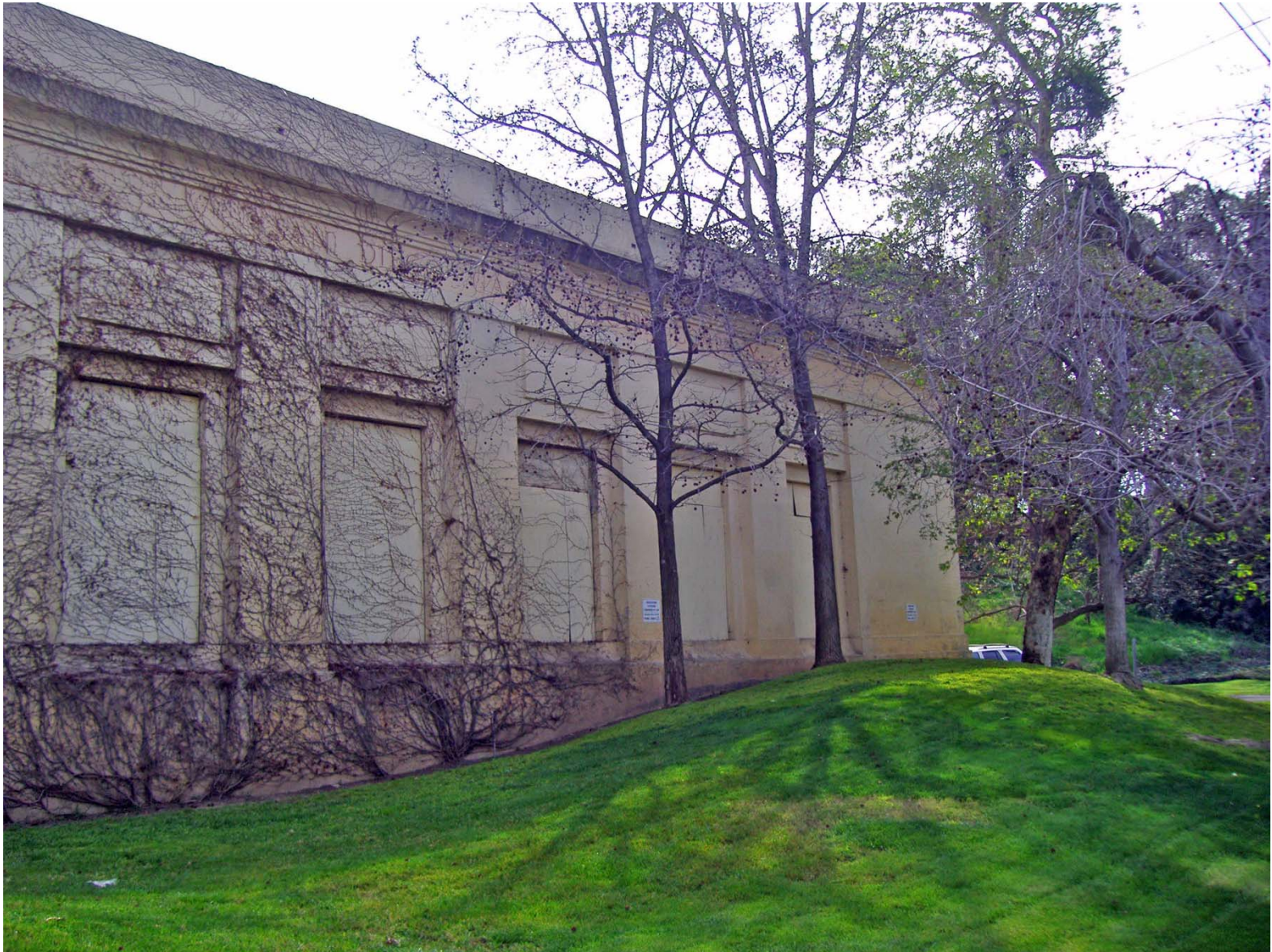
Overview of West Elevation of SD G & E Building (facing Southeast).
