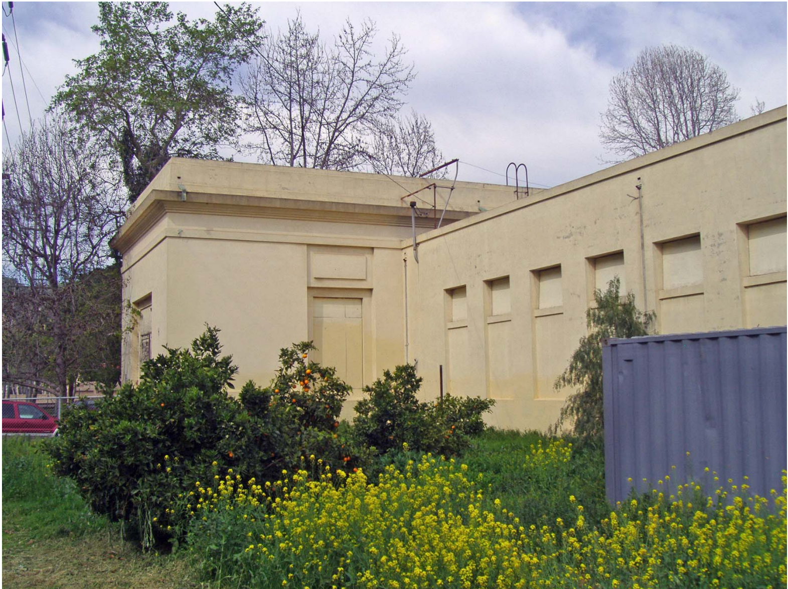
Overview of SD G & E Building from Southeast (facing West/Northwest).
