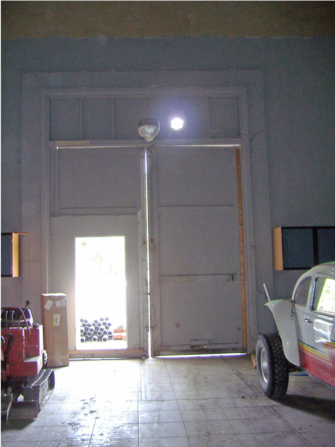
Overview of North Elevation from Interior of SD G & E Builising, San Juan Capistrano (facing North).
