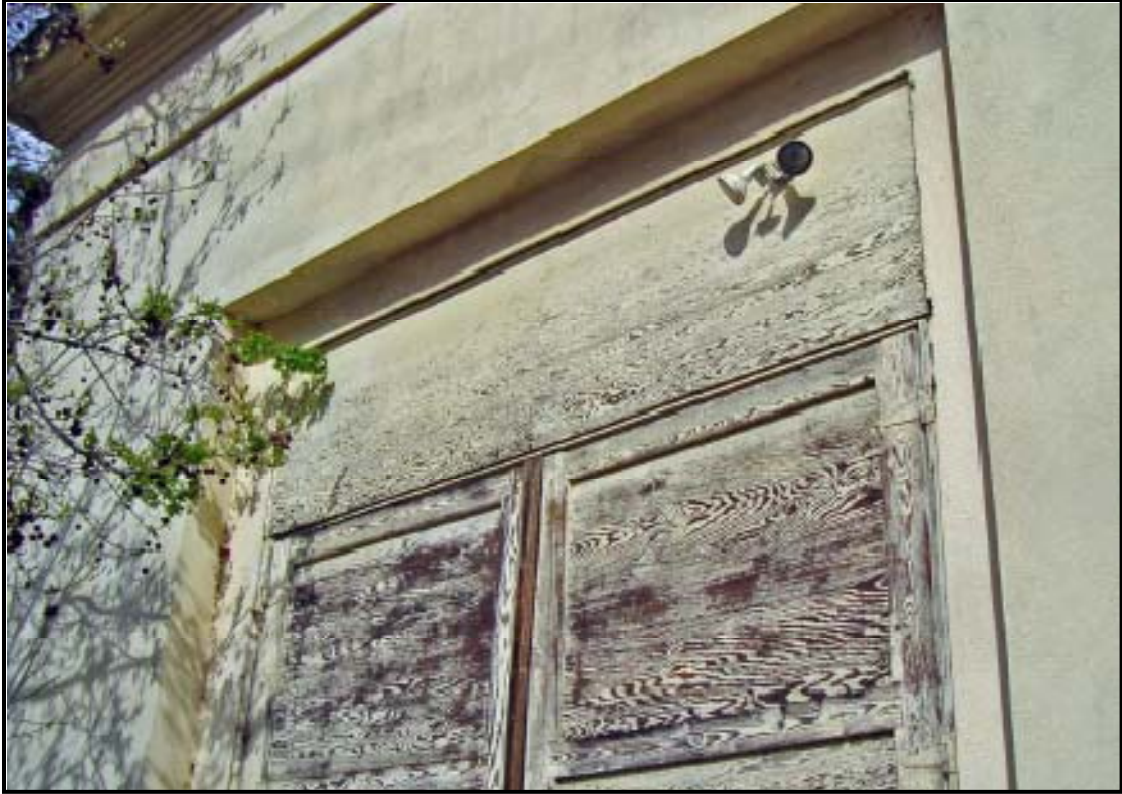
Figure 17. View of Main Entry on South Elevation of Machine Room.
