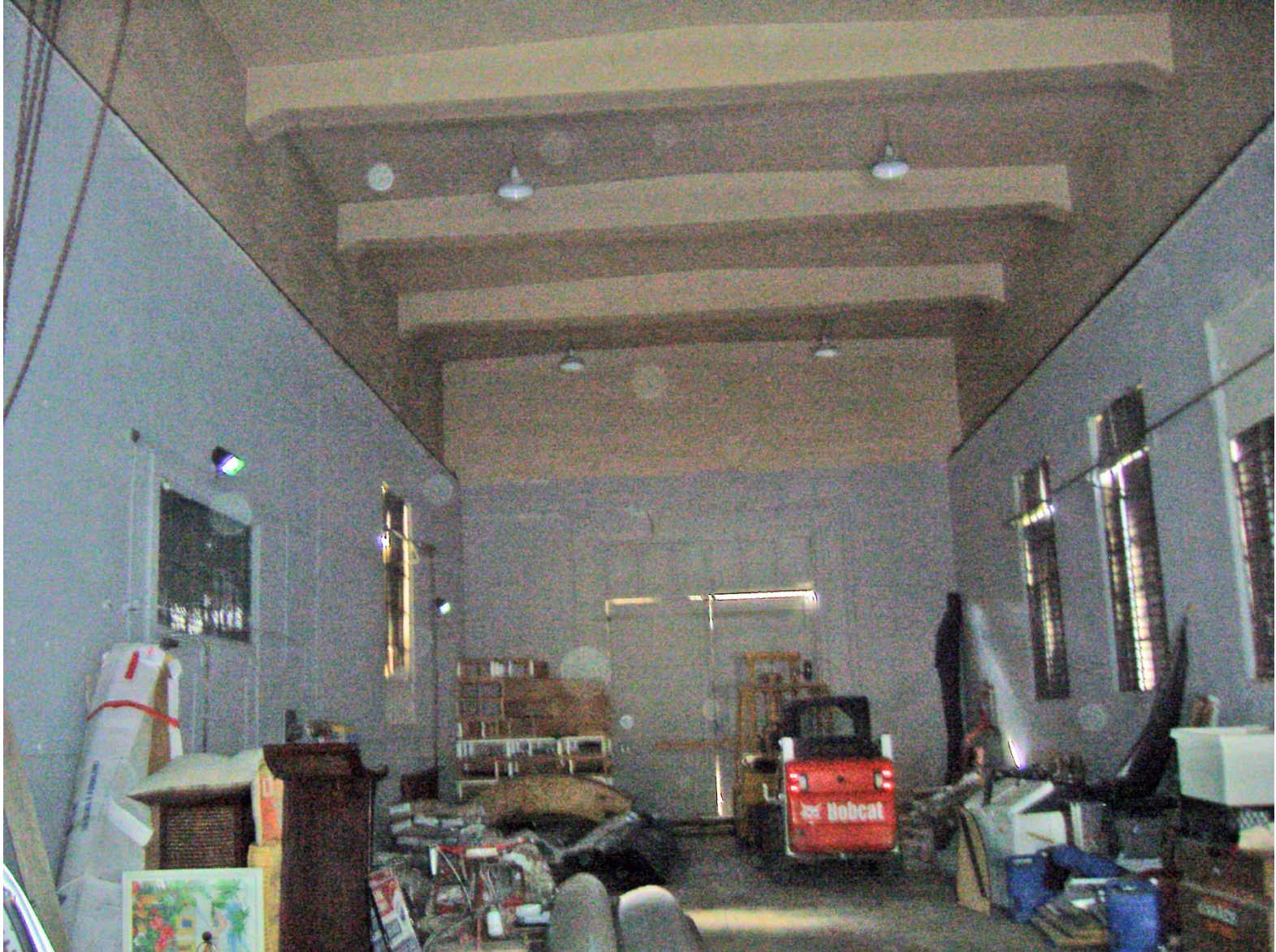
Interior of Main San Diego Gas & Electric Building, San Juan Capistrano (facing South).
