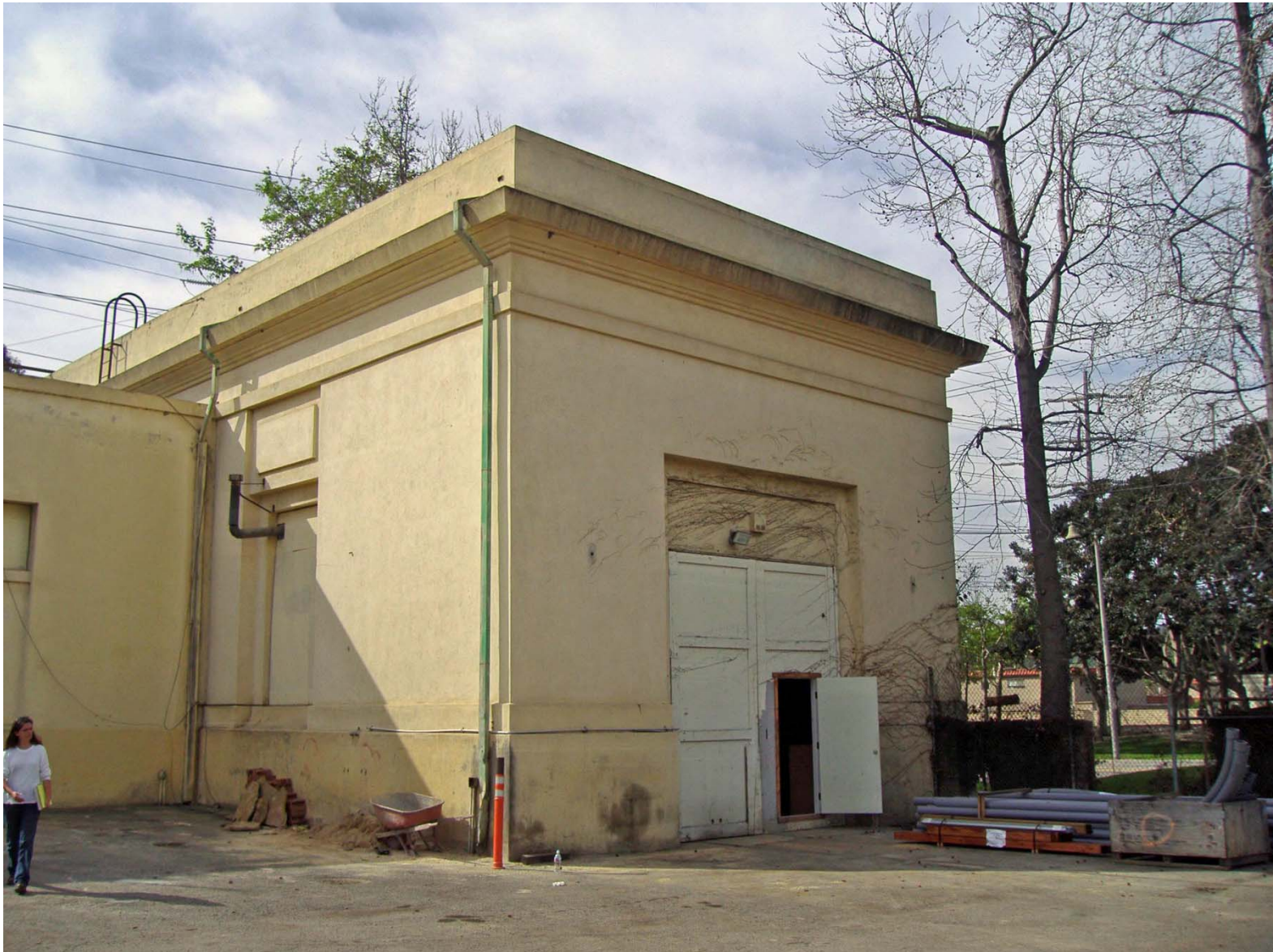
Overview of Eastern Extent of North Elevation of SD G & E Building, San Juan Capistrano (facing Northwest).
