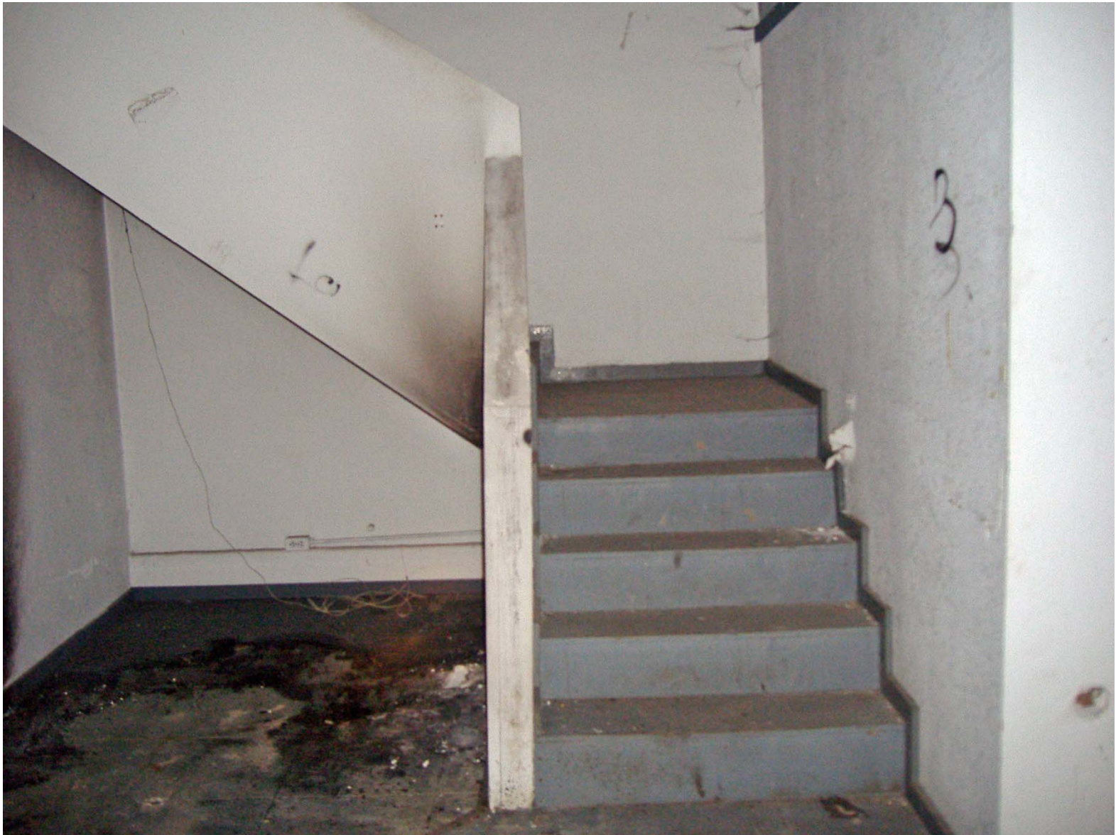
Concrete Stairway to Second Story Offices (facing North).
