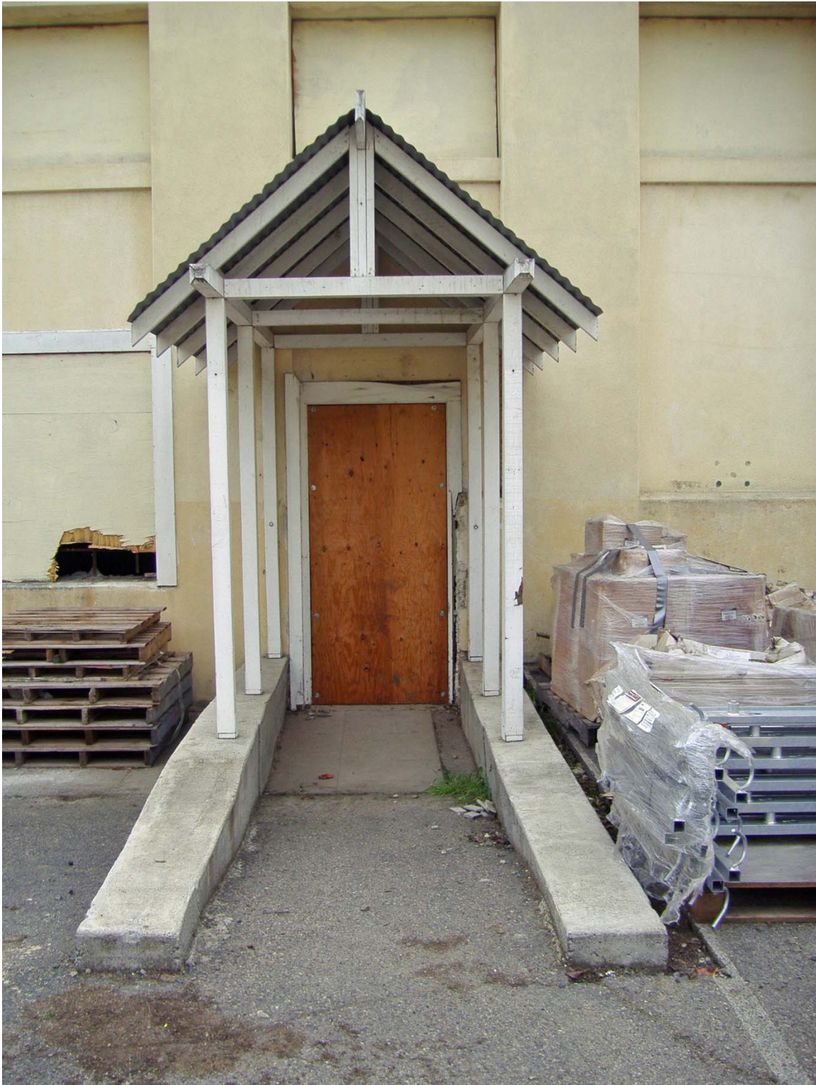
View of Accessed Doorway on North Elevation of EII (facing South).
