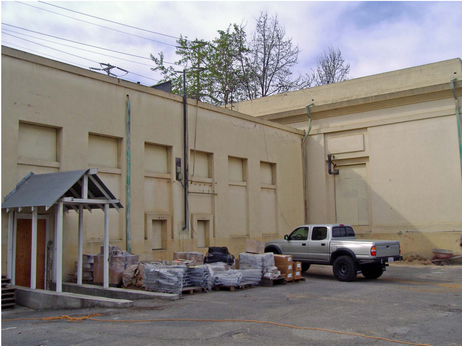
Overview fo Western Portion of North Elevation of Ell (facing Southwest).
