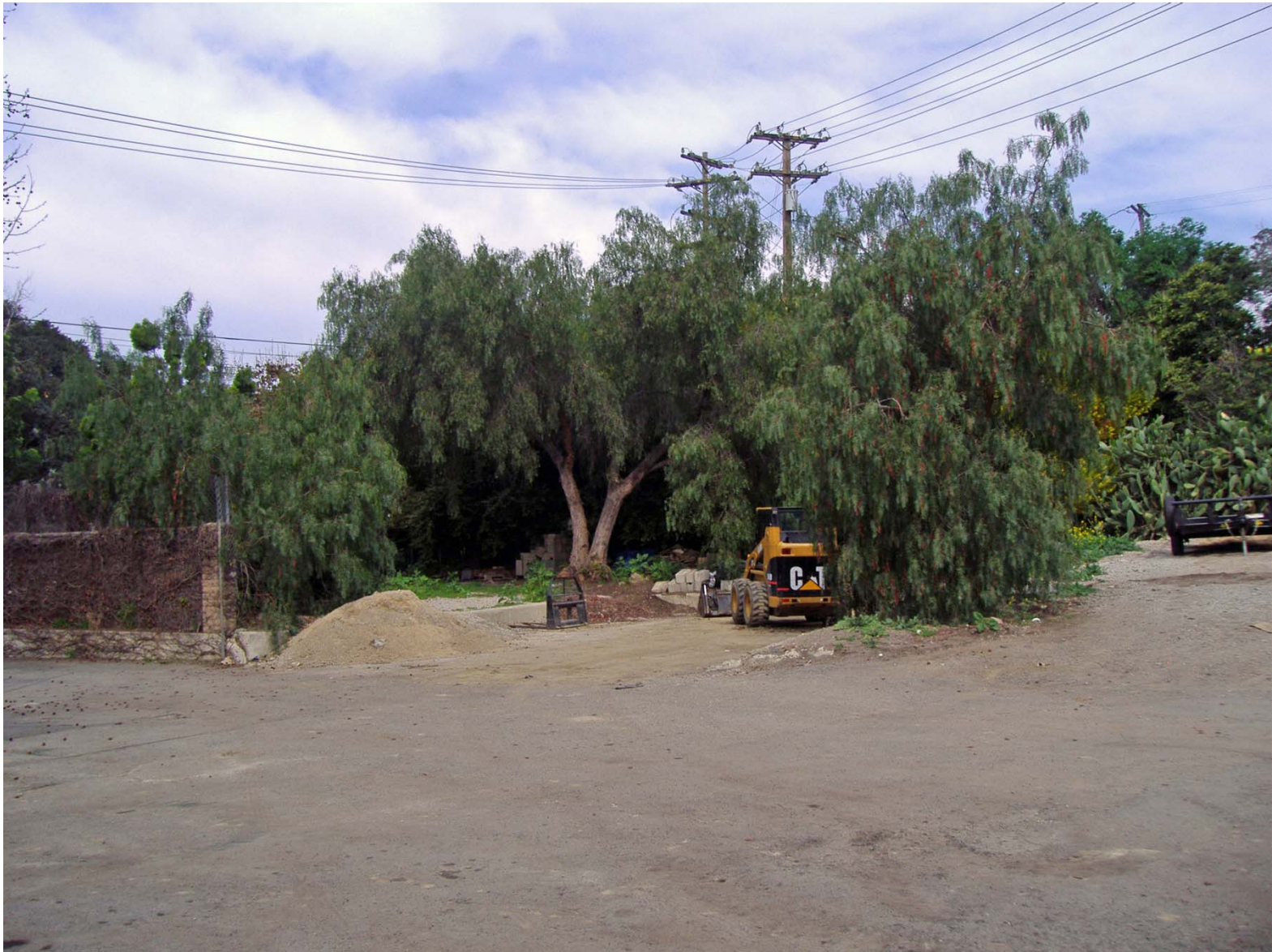
Overview of Yard Area to North of SD G & E Building (facng North).
