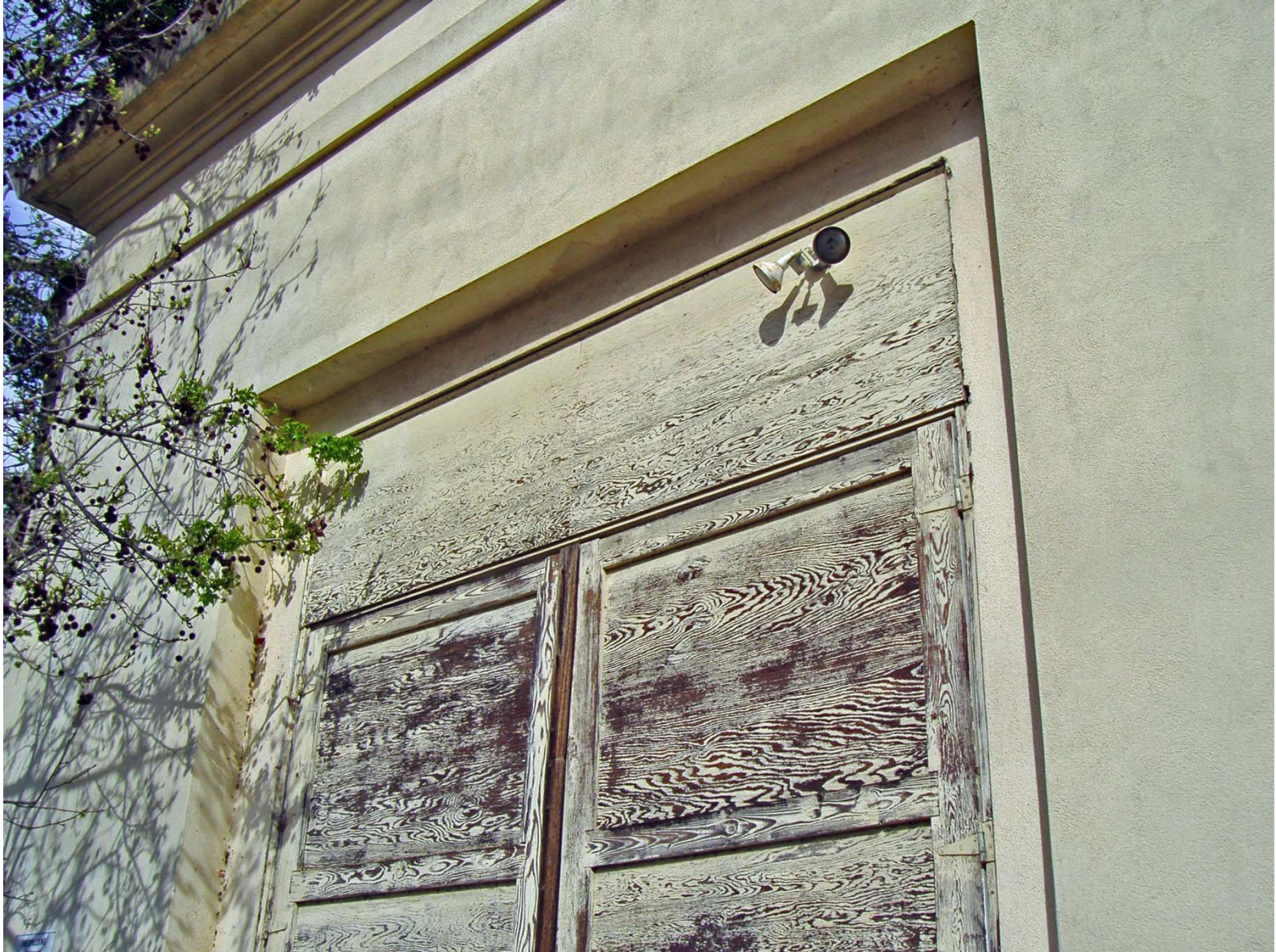
Covered Window over Bay Doors on South Elevation (facing Northwest).
