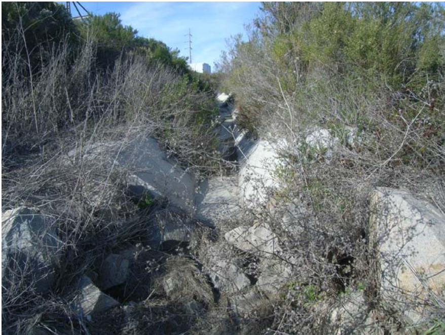
Photo 16: View of Tributary to Christianitos Creek 2 facing north. The feature was partially channelized in a two foot concrete channel.
