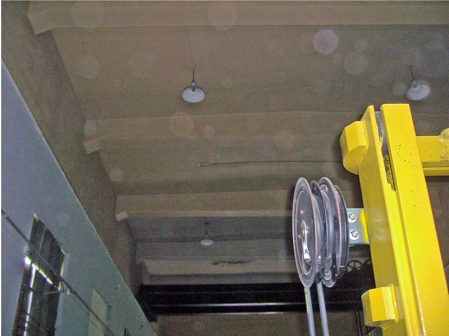
Detail of Ceiling Beams and Lighting within SD G & E Building.
